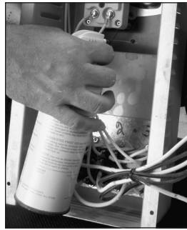
Cleaning the switch box with canned air.
