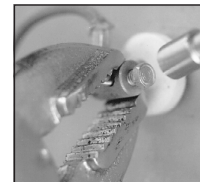
Installing the element connectors.
