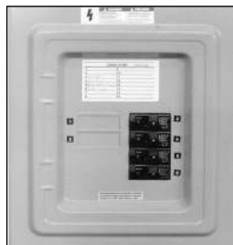
If possible, install the kiln within 25' of the breaker panel.
